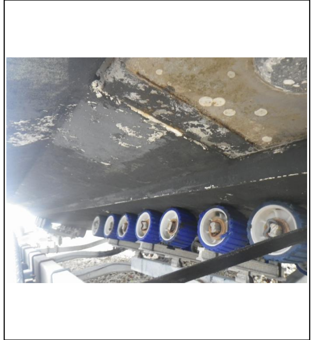
Bottom should be painted
